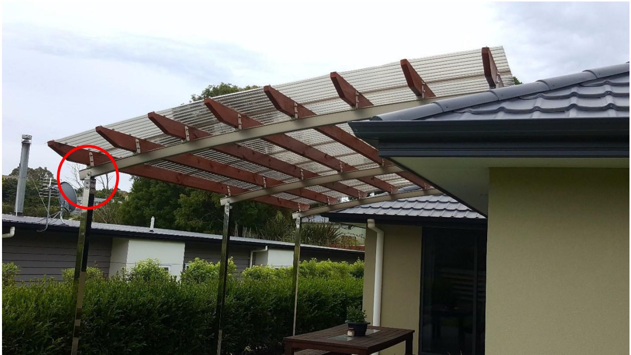
Photo 1 – showing the position of the connection within the final structure
